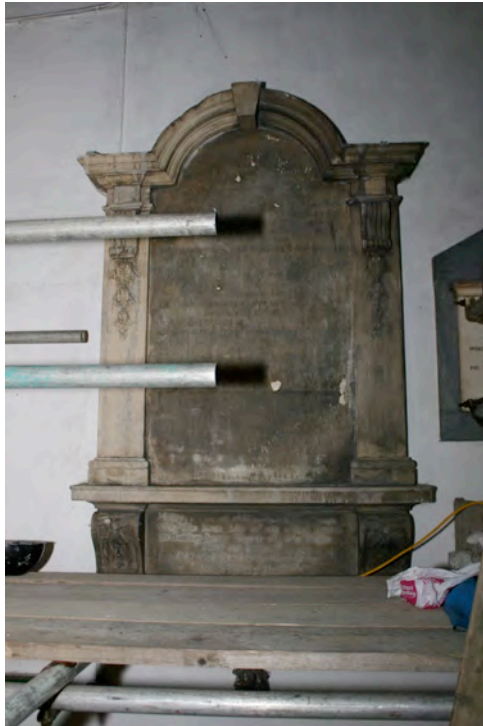
General views of the monument during cleaning, with the viewers left side partially cleaned on the left image and the right-hand pilaster during cleaning on the right. Note on this image the small, splash marks which became apparent all over the surface during cleaning with cotton wool swabs. This type of random, soiling is sometimes seen on wall-paintings and is attributable to bat urine, close to a roost.
