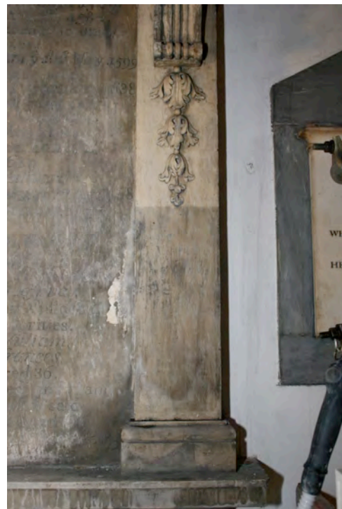
General views of the monument during cleaning, with the viewers left side partially cleaned on the left image and the right-hand pilaster during cleaning on the right. Note on this image the small, splash marks which became apparent all over the surface during cleaning with cotton wool swabs. This type of random, soiling is sometimes seen on wall-paintings and is attributable to bat urine, close to a roost.
