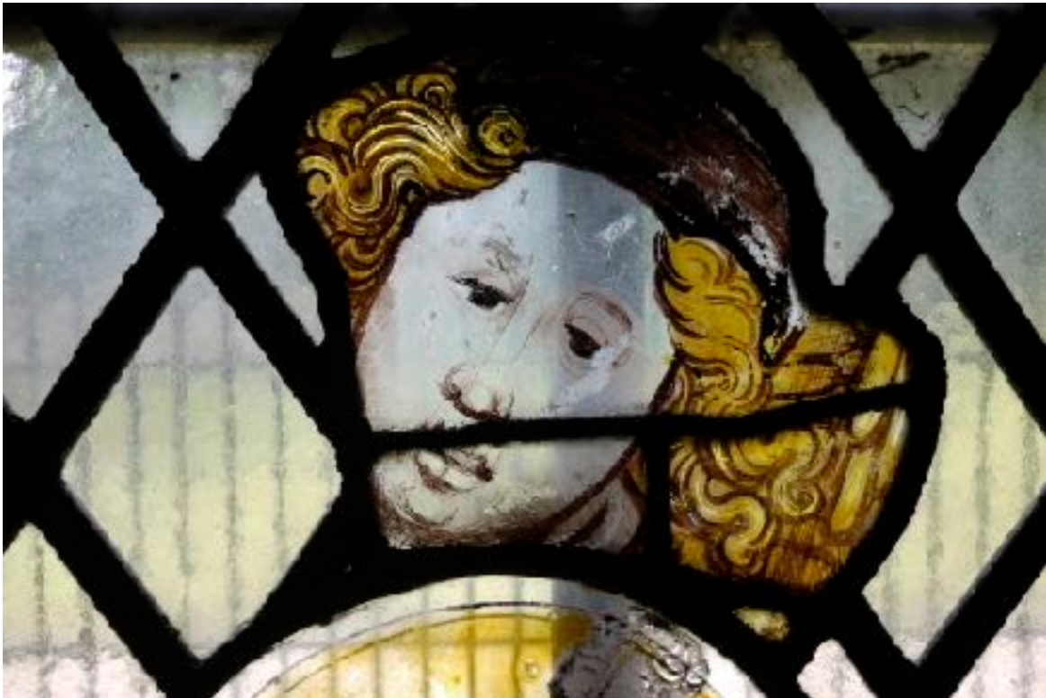
sIV 2b detail: internal fracturing visible to face of angel
