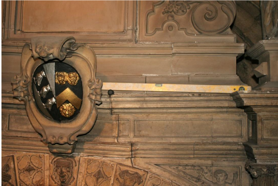
General view of the south elevation, highlighting the deformation present in the canopy, note the vertical joint has opened up from the extrados of the arch to the top bed of the cornice and has been filled with plaster to make up the moulding. The spirit level is perfectly horizontal, highlighting the discrepancy of 30mm, with a maximum of 44mm in the same place on the north elevation. This would need to be taken into consideration when re-building the canopy plumb/horizontal.
