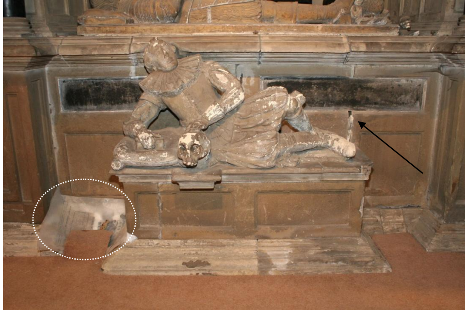
General view of the south elevation, the arrow indicates where visual access to the core of the tombchest was possible. The area circled shows where trials were undertaken to remove and replace defective mortar, being covered with damp cotton-wool and plastic to prevent premature drying, this will be monitored closely to chart the anticipated movement of soluble salts through the new mortar.
