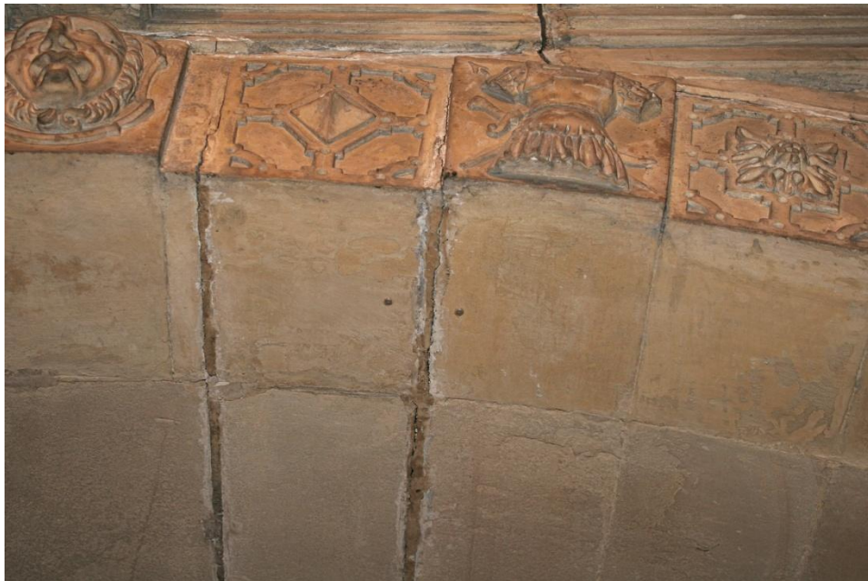
General view of voussoirs one and two to the east of the keystone, the Demec studs had closed up by 15.49mm over the course of five months from the date they were applied, with the joint now appearing tight.
