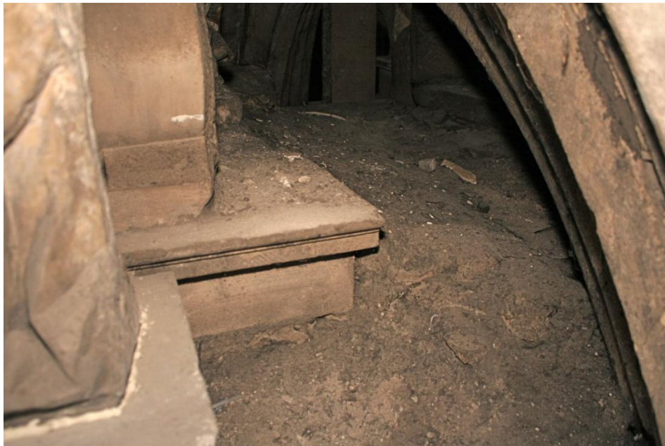
General view from the south-east corner , inside the top of the canopy highlighting the extent of rubble stonework and mortar spanning between the two elevations, adding unnecessary weight to the crown of the arch/vaulting.
