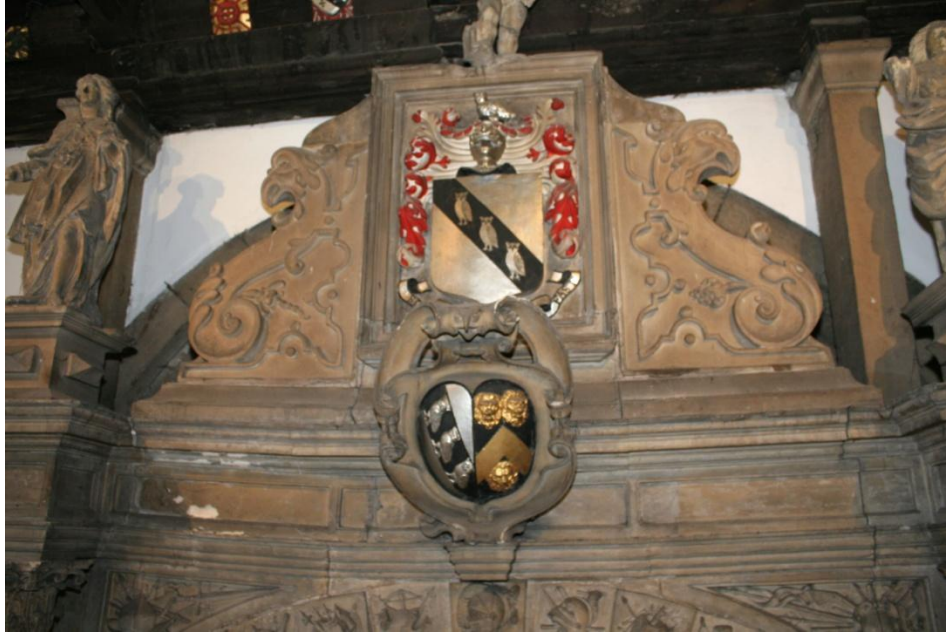
The main horizontal axes of the canopy on the north elevation, note the overall extent of deformation/sagging, note also the extent of surviving decoration and its relatively sound condition.
