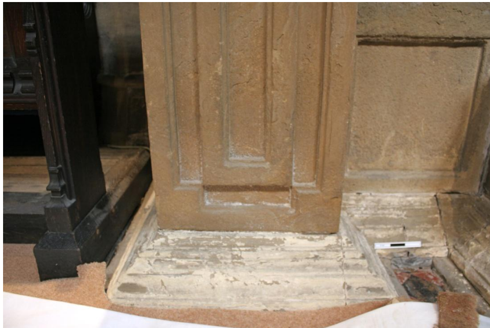
Context view of the left-hand plinth and pilaster, highlighting the loss of painted material from the plinth. Note the light-grey areas are fluffy efflorescence which should be vacuumed on a regular basis to prevent them moving in and out of solution.
