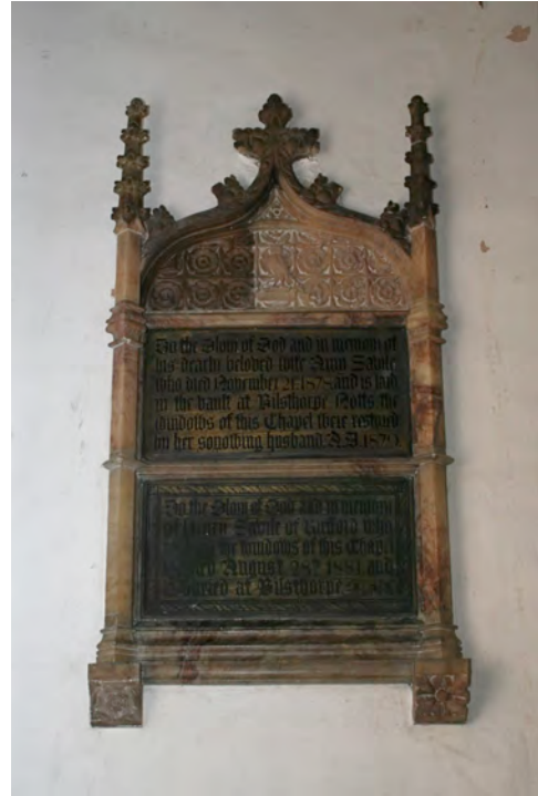
General view of the monument before and during treatment, with a cleaning contrast clearly visible to the upper elements. Note how the carved detail to the panel within the ogee arch, are completely lost due to the heavy uniform soiling.
