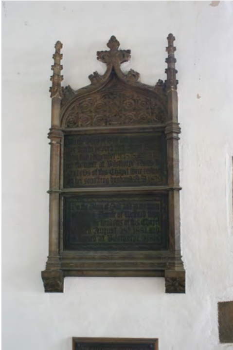
General view of the monument before and during treatment, with a cleaning contrast clearly visible to the upper elements. Note how the carved detail to the panel within the ogee arch, are completely lost due to the heavy uniform soiling.
