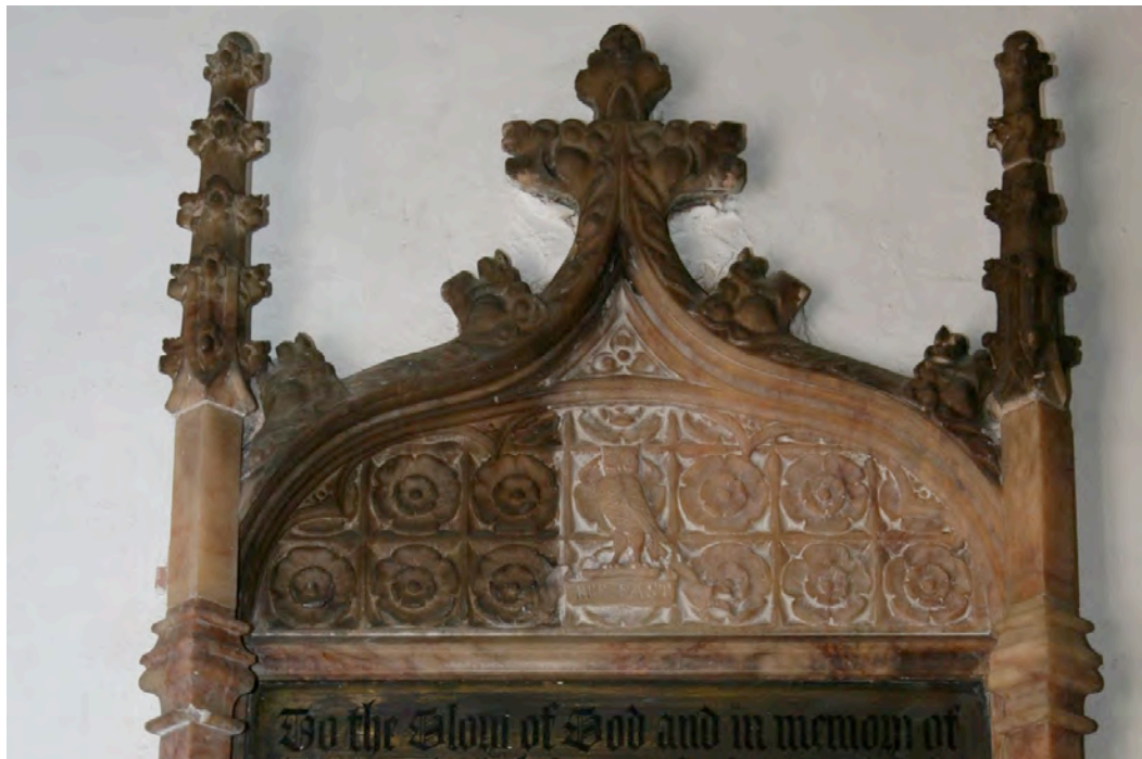
Detail of the repeat foliage decoration incorporating the Savile family motto, note how the rich veining within the alabaster has been restored visually.
