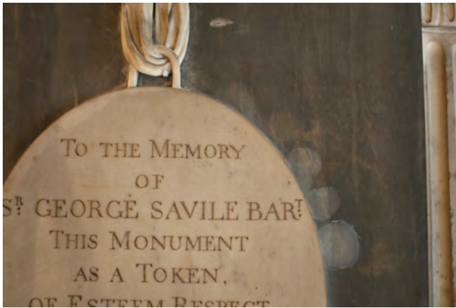
Cleaning trials in progress around the perimeter of the elliptical inscription panel, note how heavily soiled the dark-grey background panel was prior to wholesale cleaning.
