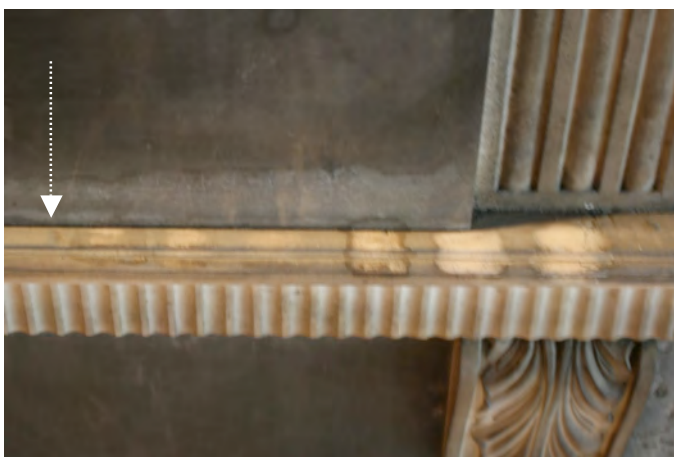
More cleaning trials to a discrete, heavily soiled area of the white marble, with trials starting at the far left-hand side (indicated) with more gentle, volatile materials, gradually increasing in strength to the abrasive paste at the far right-hand side.
