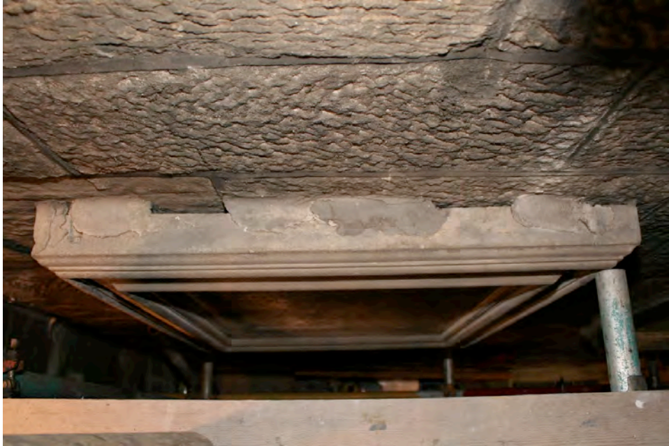
The top bed of the monument showing the location of restraint fixings securing the top moulded element to the wall. Note the small air gap between the tooled walling and the rear surface of the moulding, which will have prevented penetrating moisture transferring into the inscription panel. Note there were no signs of iron staining or corrosion jacking from beneath the mortar so it was left.
