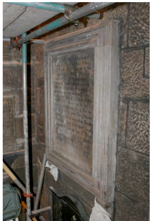
The left-hand image showing paper towelling in place, dampened with the cleaning solution, which keeps it at the surface, rather than saturating the stonework. The right-hand image shows the level of cleanliness achieved on the moulded border, with just the corbels left to clean.
