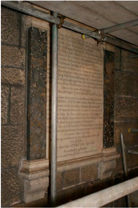
General view before and after treatment, note again the brown cast to the light coloured marble on the left-hand 'before' image and the marble looks fresher after cleaning.
