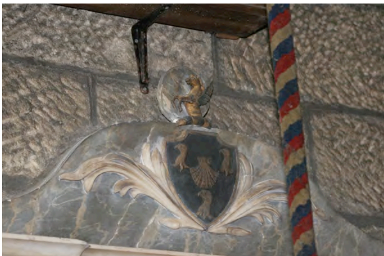
Context view of the pediment, note the veining is visible in the pediment once again, although the surface polish has long since gone, again possibly due to direct sunlight playing over the surfaces, with heating/cooling cycles setting up surface condensation over a prolonged period of time. This is a clearly a decorative marble and not that robust evidenced by the pilasters.
