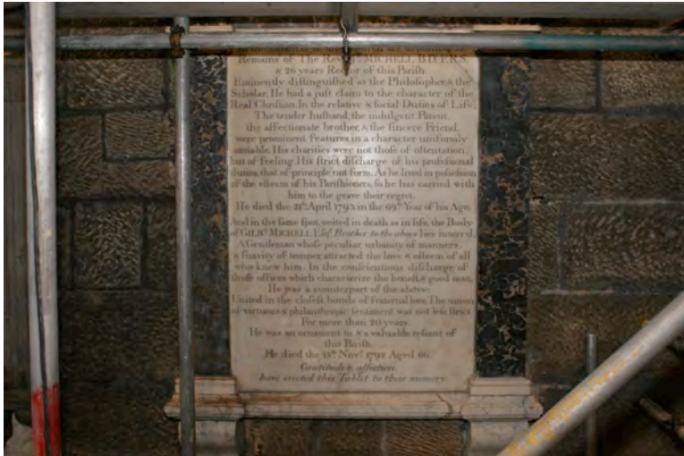
A cleaning contrast to the inscription panel, with the right-hand side having been cleaned from top to bottom.
