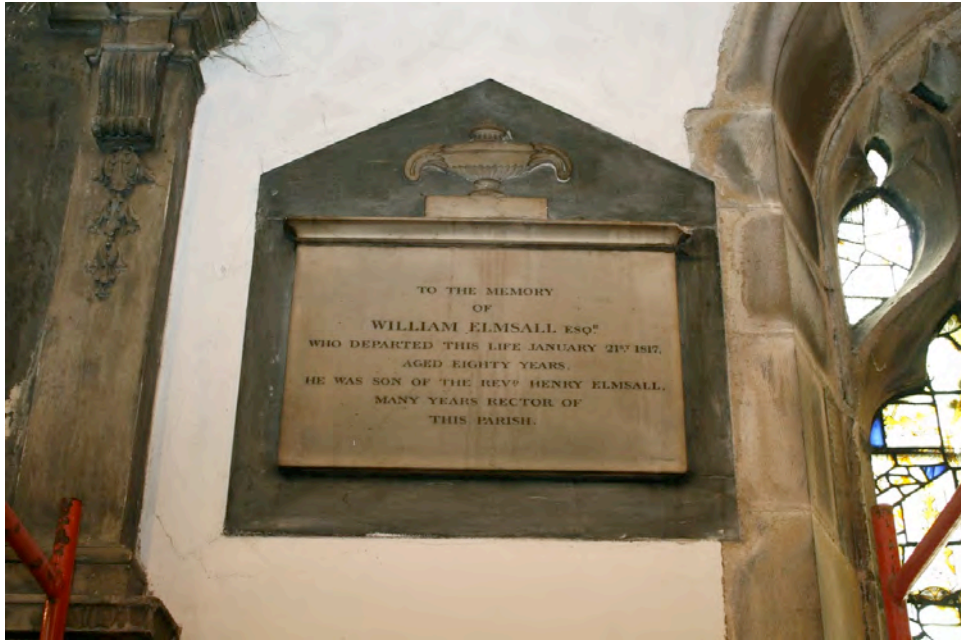
General view of the monument before treatments, note how the inscription panel in particular looks uniformly dirty.
