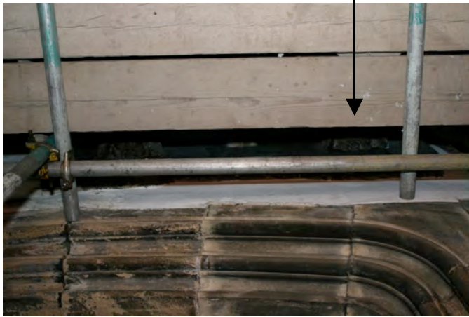
General view of the underside of the monument from floor level, before cleaning. Despite being in shadow, the foliated right-hand corbel is black. Note the levels of soiling to the moulding voussoir of the arch beneath.
