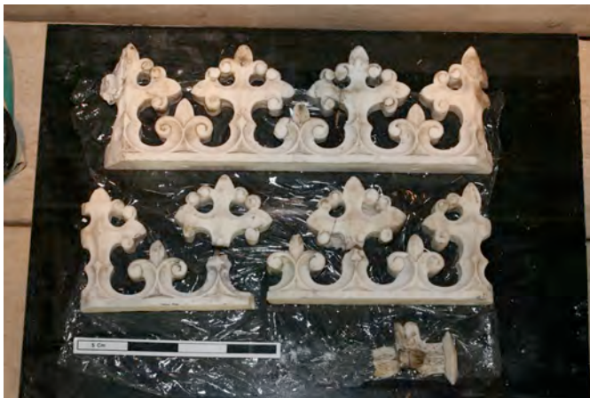
The loose bratishing sections after cleaning and before re-joining broken sections, prior to re-fixing. The bratishing was re-fixed with Polyfilla.
