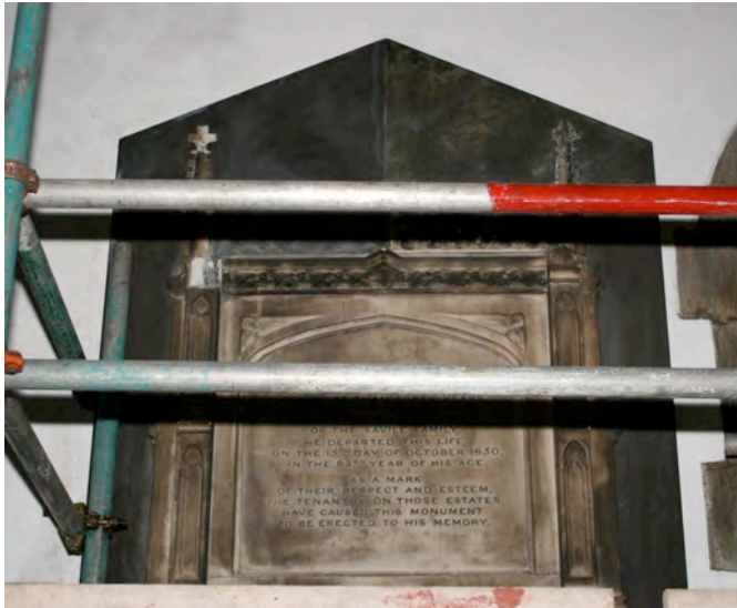
General view of the monument before any treatments. This monument is difficult to photograph in free space. Note how dirty the background marble is and appears to be a dark-grey material. Note the monument is situated immediately above the recess which is believed to have had a solid fuel stove within it historically.
