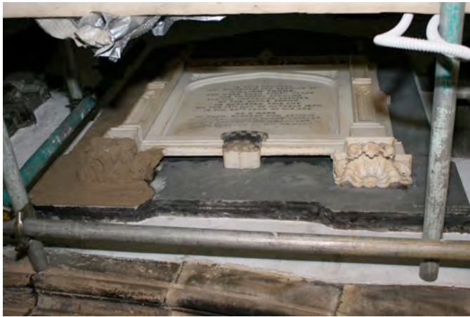
A similar view with the boards peeled back. The right corbel is clean but still displays a brown cast. The left corbel and flat background are covered with the poultice prior to removal.
